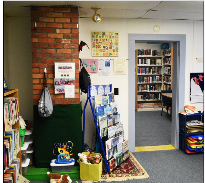
Figure 26: Exposed chimney in Children's Room
