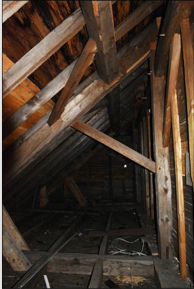
Figure 39: Unaltered southeast eave
