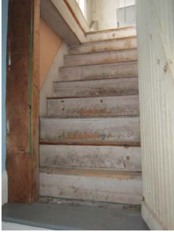
Figure 58 – Steep, enclosed stair at top of open stairway leads to 3 rd floor
