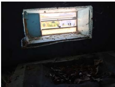
Figure 61 – louvered vents in crawlspace should be fitted with insulated covers for use in the heating season
