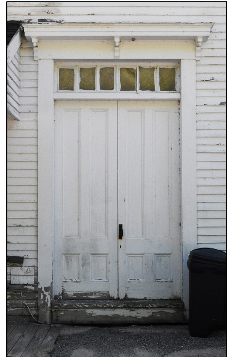
Figure 20: Central door at northwest elevation
