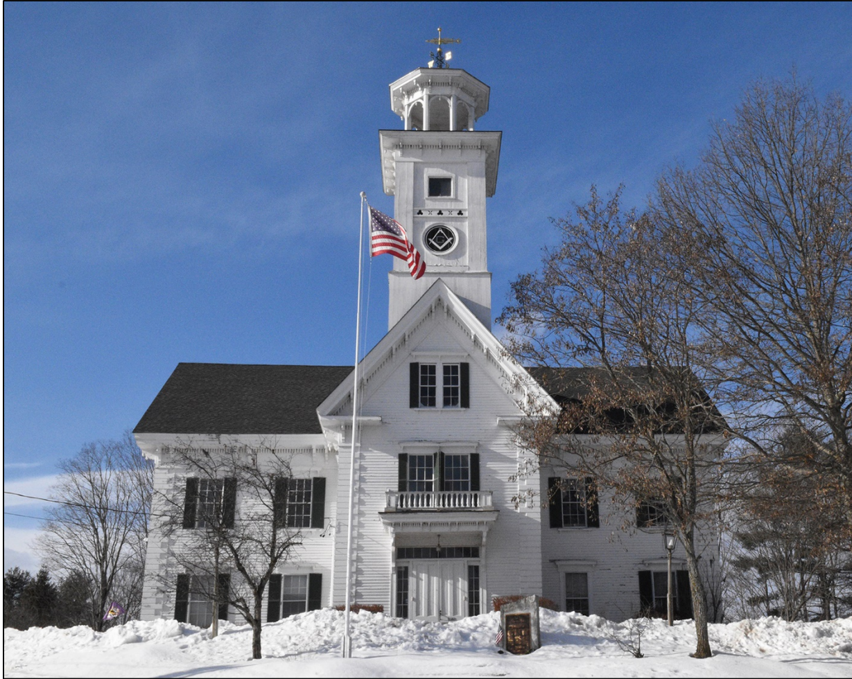
Figure 13: New England Masonic Charitable Institute facing northwest.
