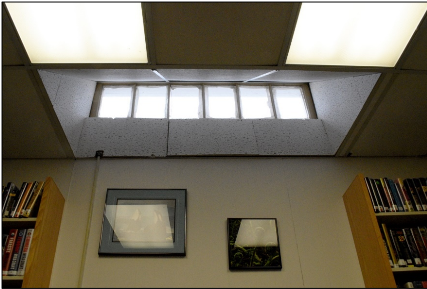
Figure 25: Transom window above former door
