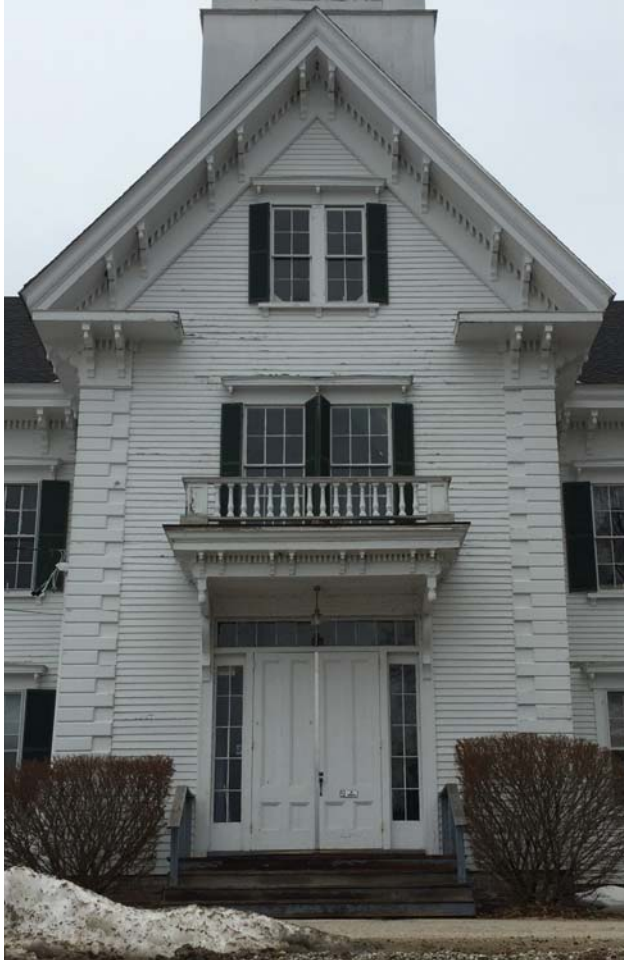
The Centered Gable Entry at the Southeast façade of the NE Masonic Charitable Institute
